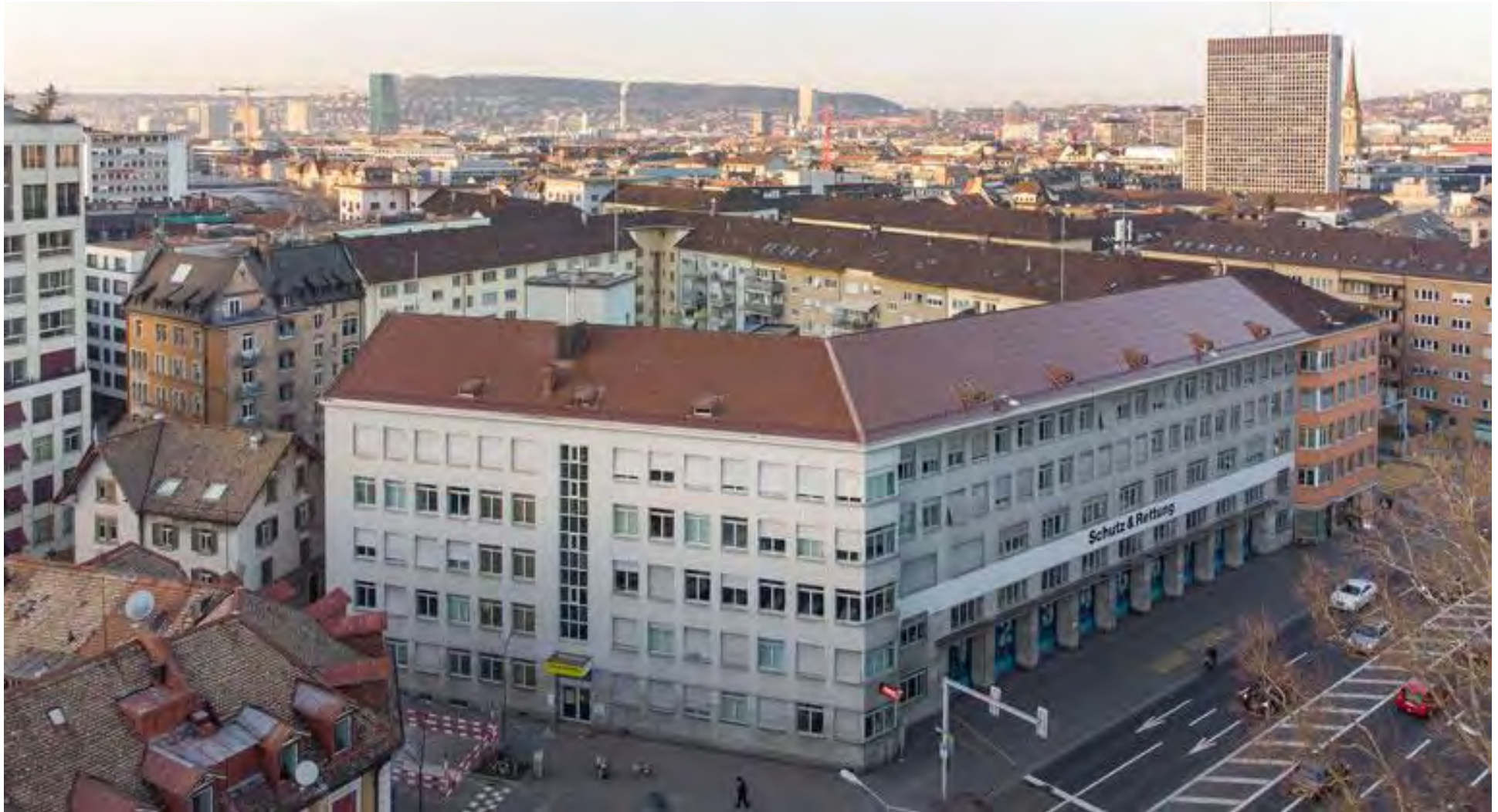
Zürich 76 kW BIPV-Anlage in Terracotta Rost Suntechnics 2021
